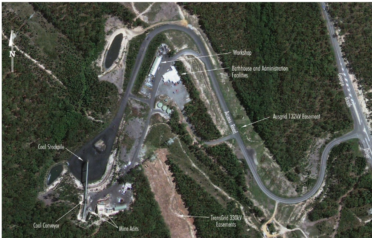
Plate 1 – Existing Tasman Underground Mine Pit Top
