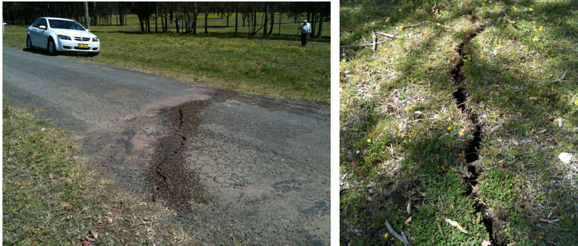
Figure 3.11 Photographs of Typical Surface Cracking in SMP Area 1 at the Abel Underground Mine (50 metres to 100 metres Depth of Cover)
