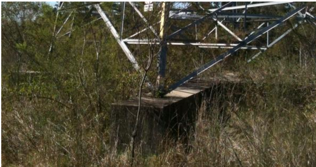
Photos 1 & 2 – Typical “cruciform footing” at base of towers
