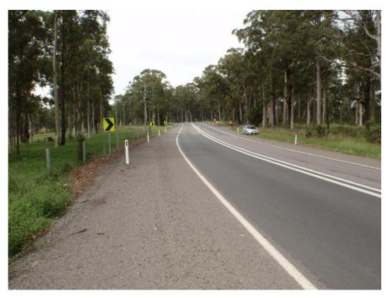
Photo 5 No. 1395 Guide Posts Restricting Available Shoulder Width
