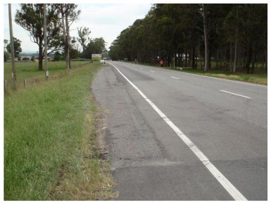
Photo 20 Insufficient Right Turn Shoulder Widening
