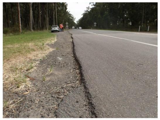
Photo 2 No. 1332 Northbound Pavement Edge Drop Off
