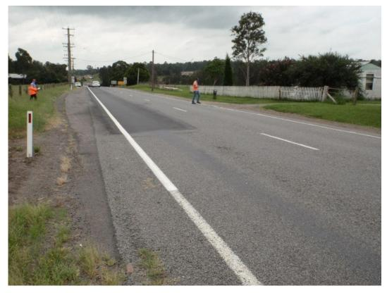
Photo 27 Right Turn Shoulder Widening Doesn't Cover the First Driveway
