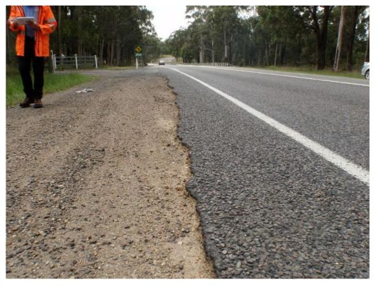
Photo 1 No. 1332 Southbound Pavement Edge Drop Off
