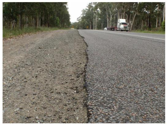
Photo 4 No. 1353 Southbound Pavement Edge Drop Off
