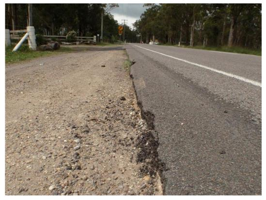
Photo 16 No. 1424 Southbound Pavement Edge Drop Off
