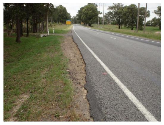
Photo 21 Edge Drop Off and Left Turn Tyre Tracks
