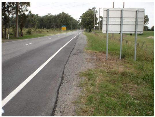
Photo 22 Rehabilitation Works stop in Shoulder and Sign in Clear Zone
