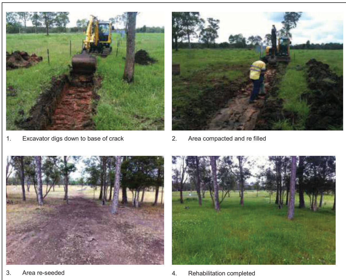
Figure 12: Typical Process for Rehabilitation of Surface Cracking
