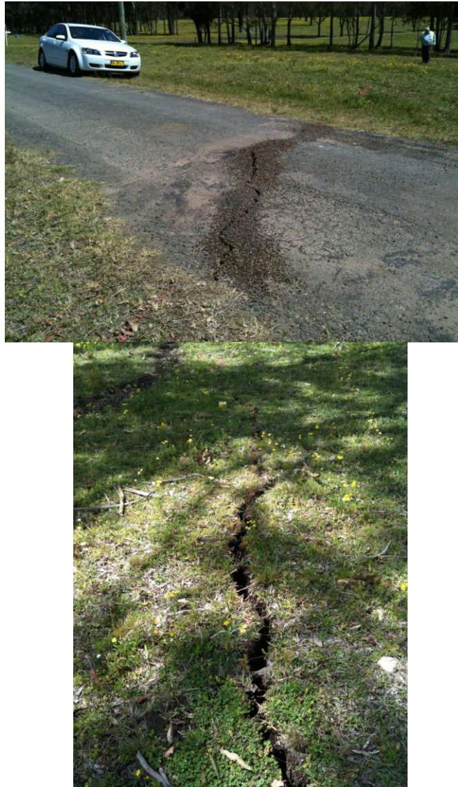
Plate 4 Typical Surface Cracking at the Abel Underground Mine (50 metres to 100 metres Depth of Cover)
