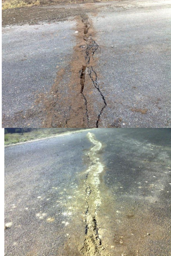
Plate 6 Impacts Observed Along Charlton Road at the Beltana No. 1 Underground Mine
